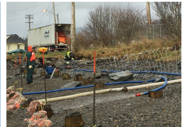
Figure 17: Contractors training in shoreline flushing.
