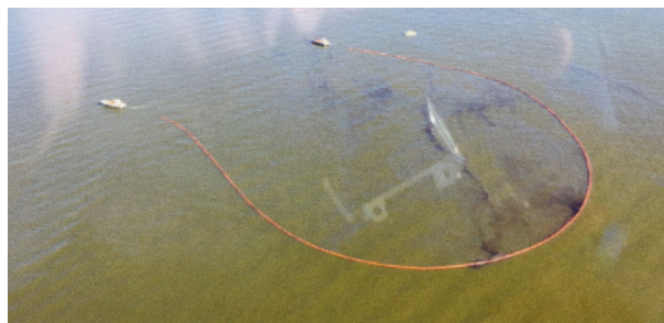
Figure 12: Boom deployed in a U-Sweep to collect oil for recovery.
